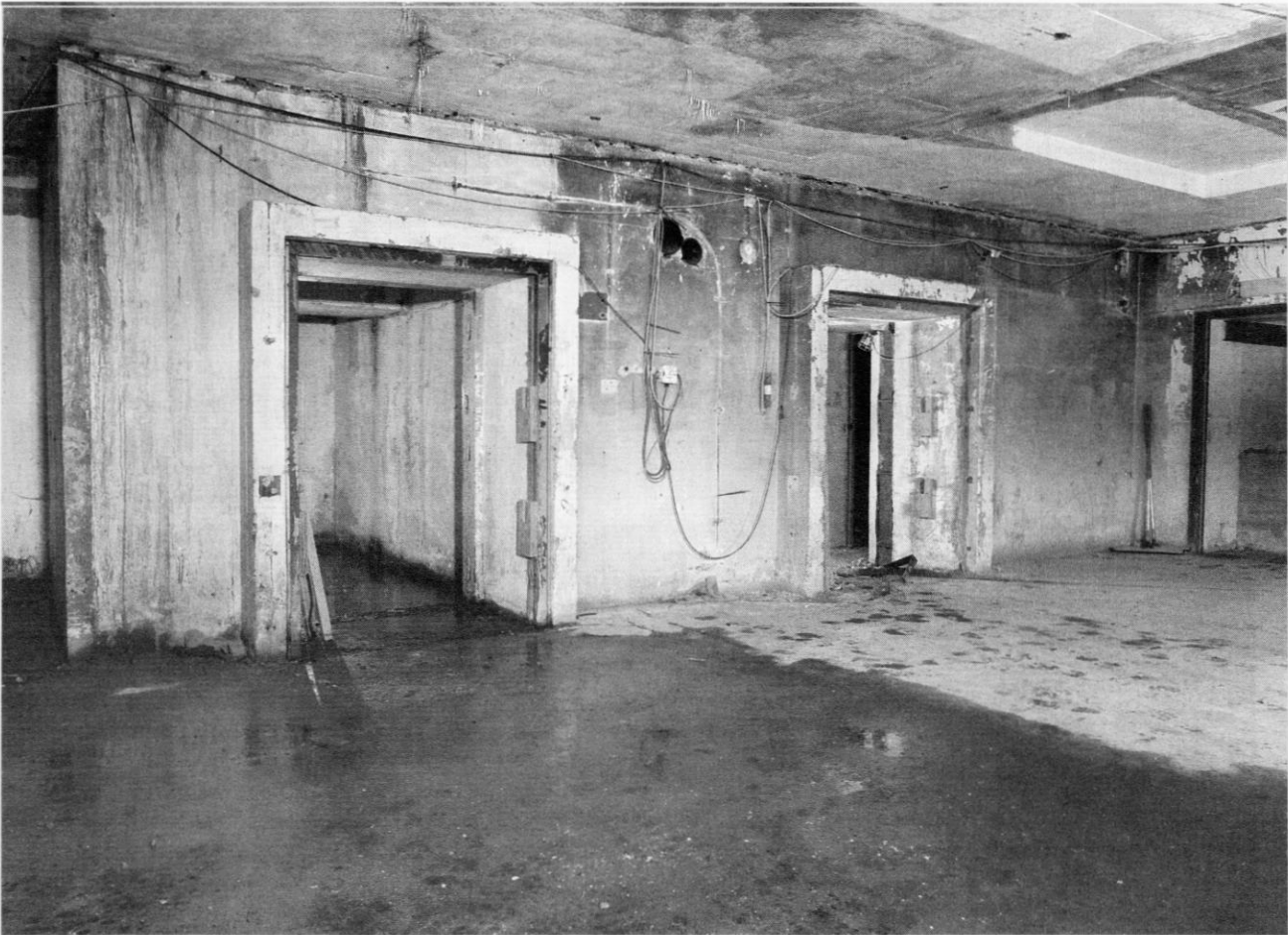
Access to the lift from the basement to the upper floors. Photo by Nick Catford
